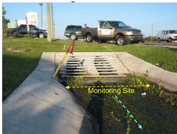
a. Transition from vegetated swale to lined ditch
