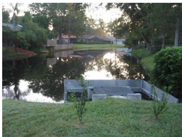
a. Outfall structure from lake system to Channel 5
